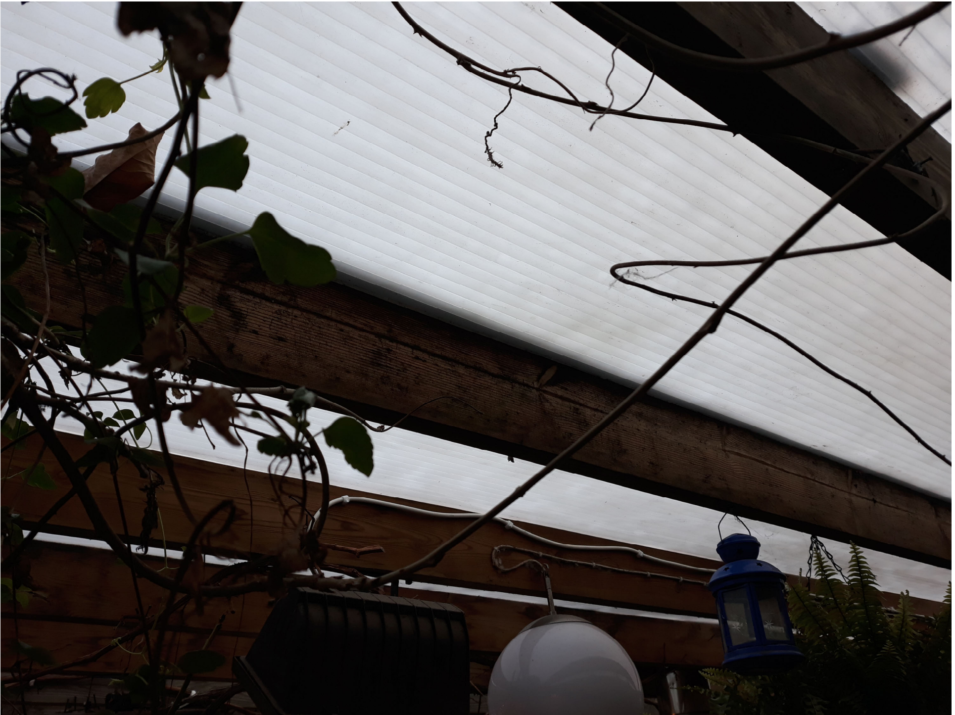
10. Roof of Outdoor Seating Area
