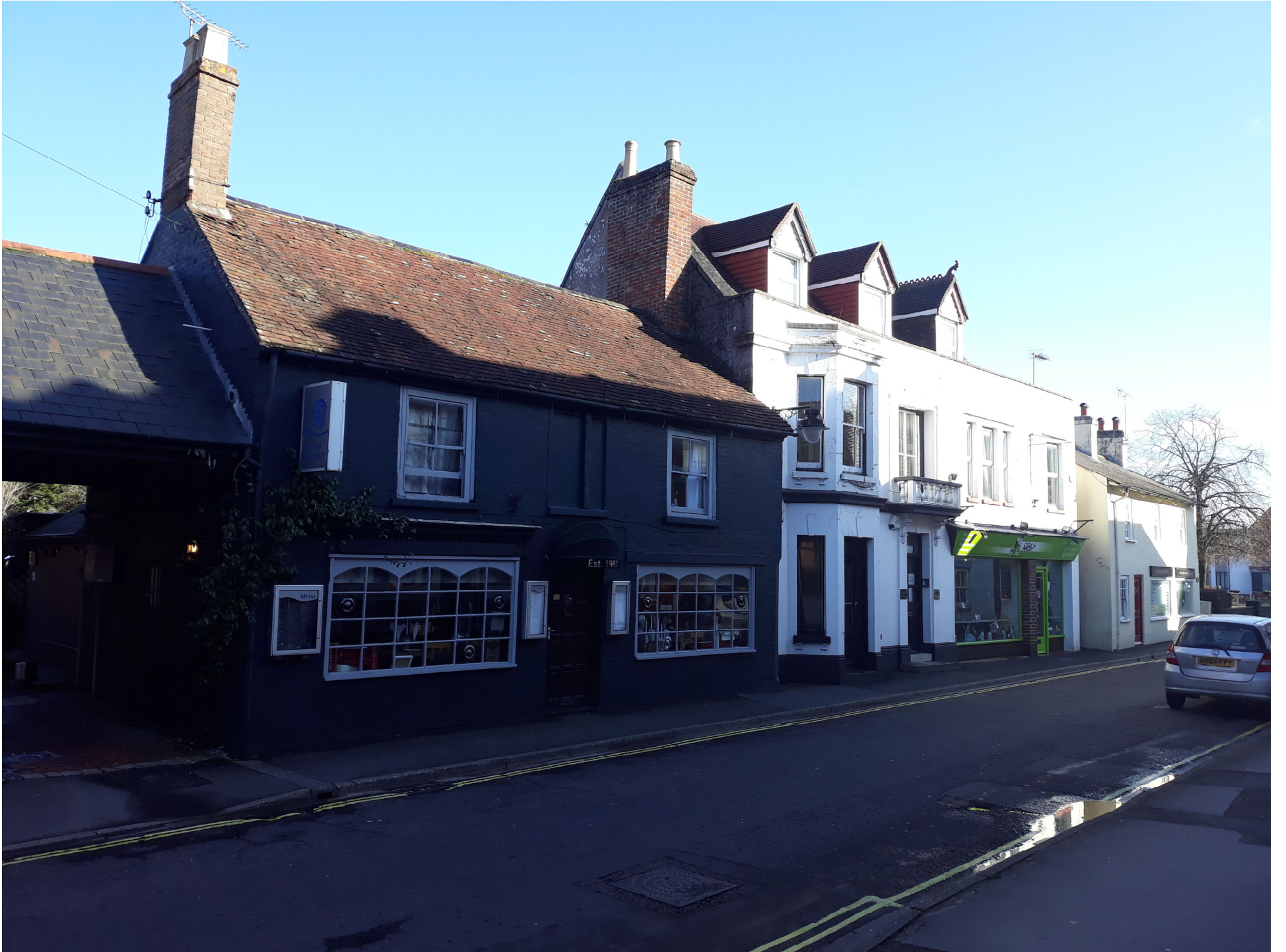
2. Front of Premises
