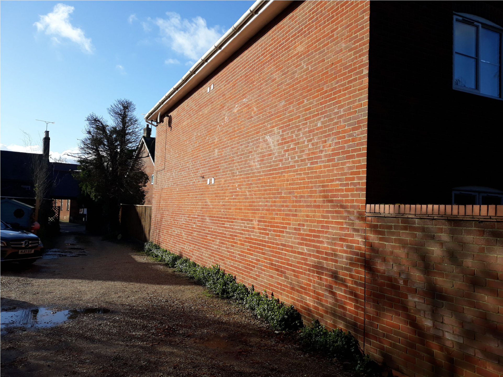
5. Car Park and Elizabeth Court Properties
